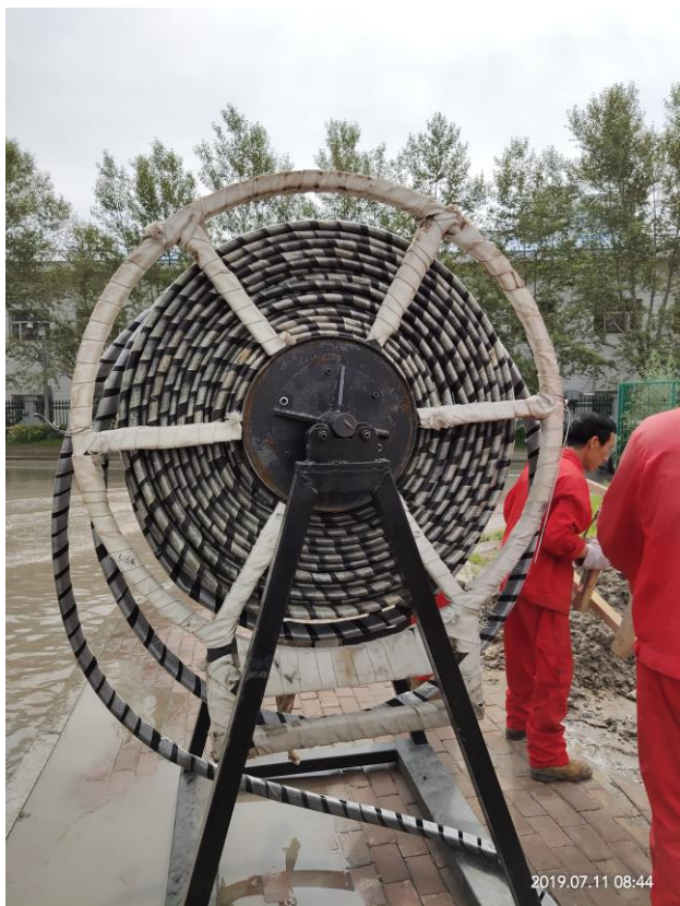
Oil Pipe DN76, 20km, Daqing Oilfield
